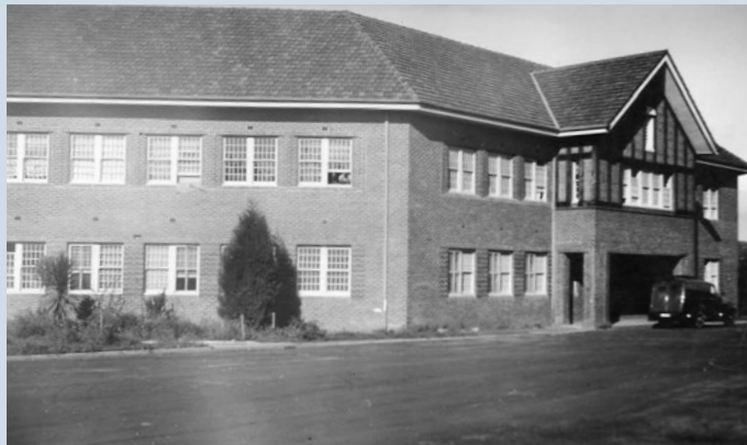
This page : Photographs taken during and post-construction of the Larundel Hospital from 1938 – 1942. Images from Public Record Office Victoria VPRS 10516/P0002/002 Opposite : Women's Auxiliary Australian Air Force poster.
