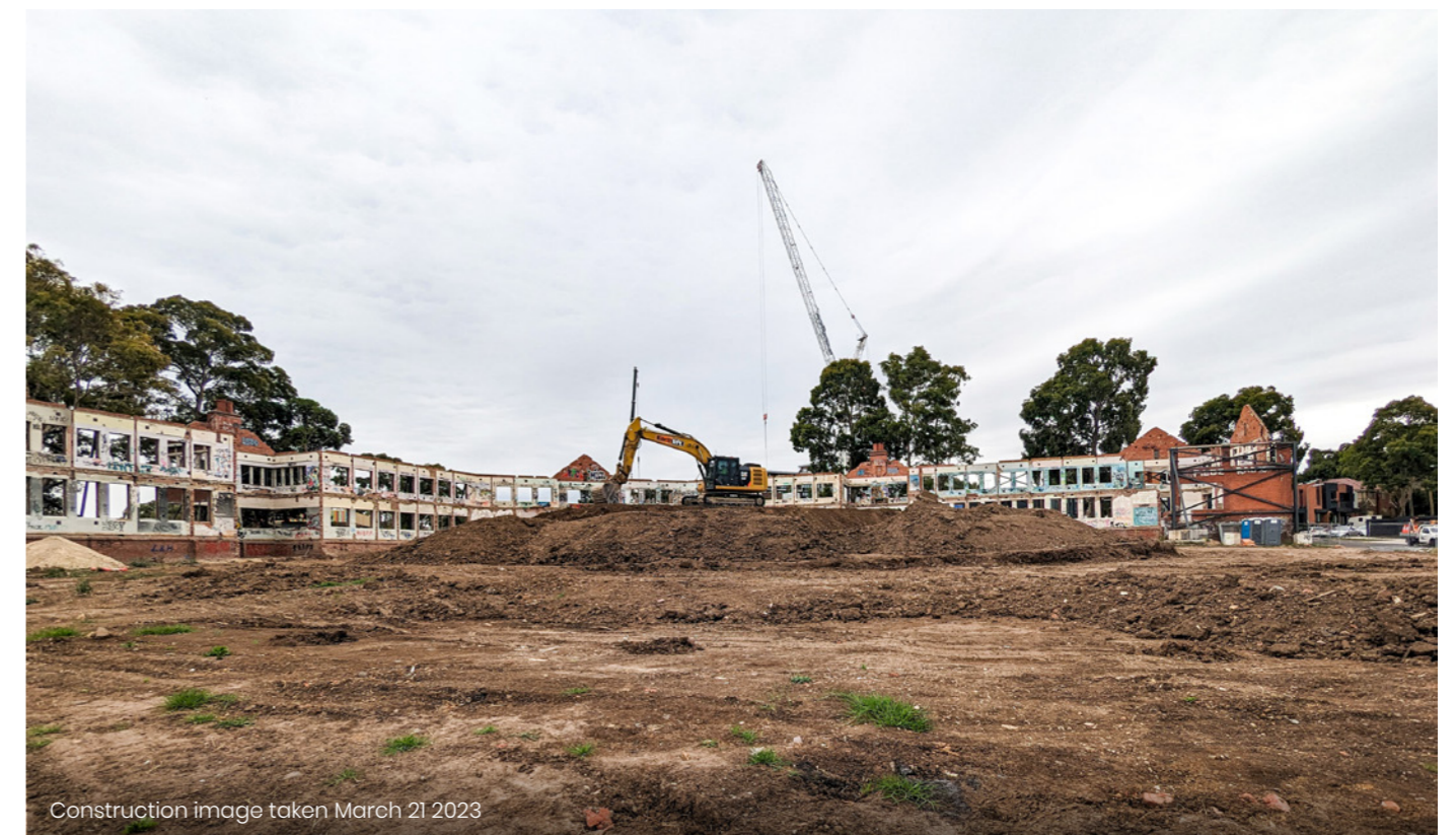
Construction image taken March 21 2023
